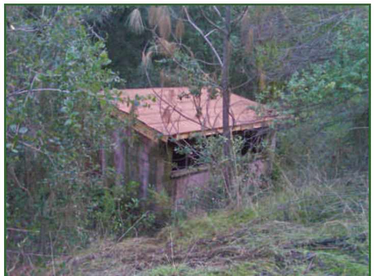
Finished roof over cinderblock restroom—GYHS
