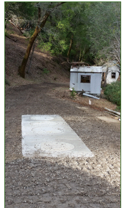
Septic access in roadway beside Texas cabin.
