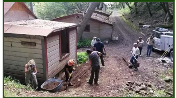
Moving dirt away from a wooden structure.
