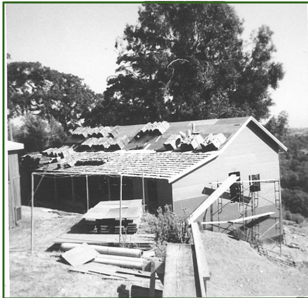
Roof going on the new Pine Ridge visitor center Photographer unknown.
