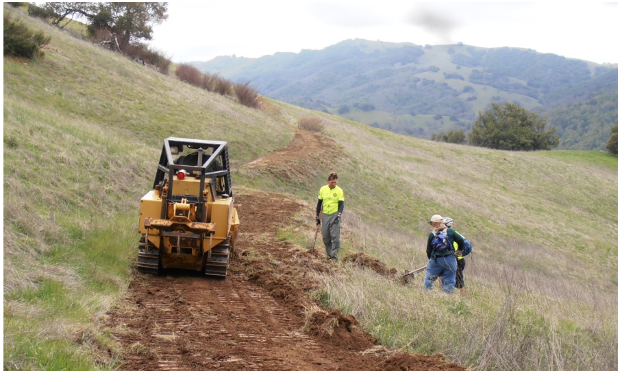
Sweco tractor working on Bowl Trail near Willson Camp. Photo by Paul Liebenberg
